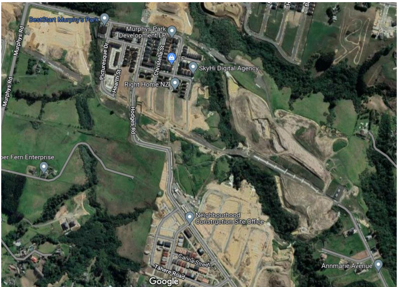
Figure 7 Recently constructed local road network
